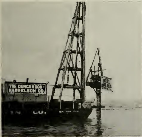
View of Barge and Column with Platform for Diamond Drilling.
